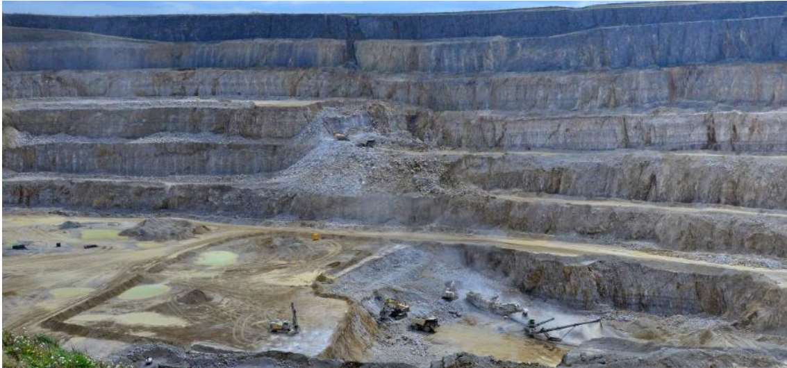
Dowlow limestone quarry in the Peak District, UK. The quarry has an area of about 0.5 km 2 and in 2021 the lowest point was some 100 m below the original land surface, but no conduits or caves have been intercepted and there is no groundwater inflow from the quarry faces. Photo by Tony Marsden.
