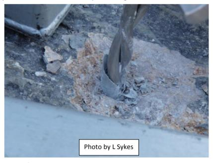
a potential related topic as to whether naturally faults and joints in limestone also have micro fractures associated with them due to the earth movement.) Images of the holes from which the Bolt Products anchors have been extracted indicate more than surface spalling has occurred.
